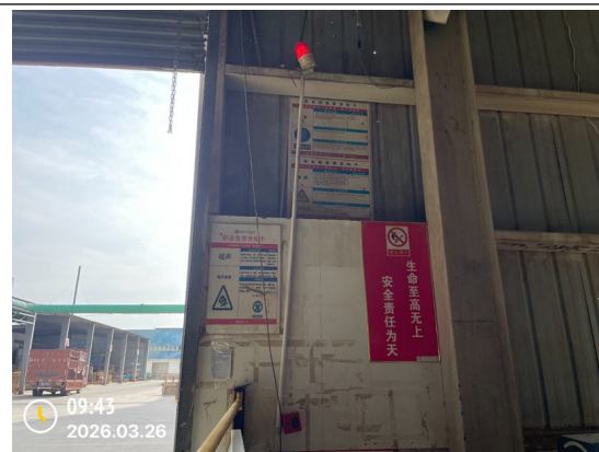
Fire alarm testing
